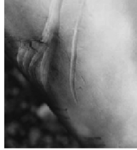
Figure 2. Example of dent on pipe.
